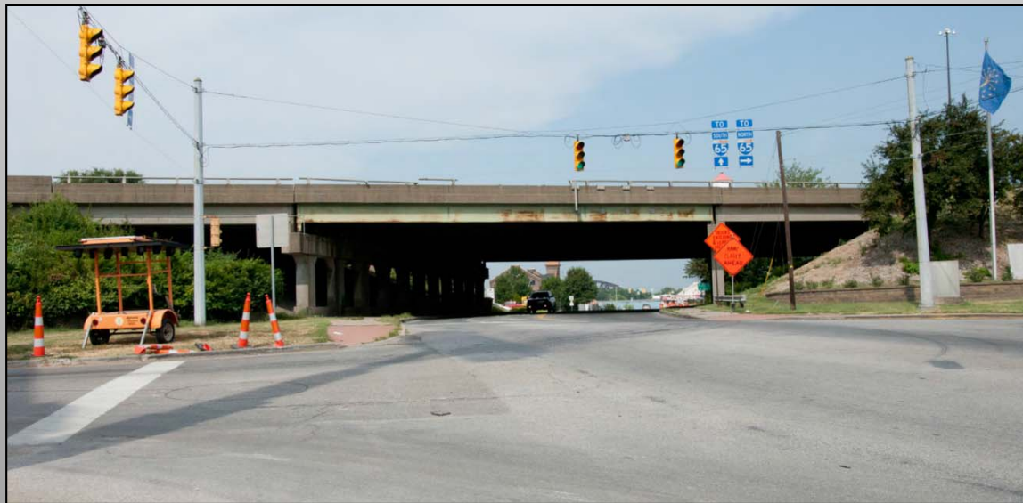
Court Avenue Existing
